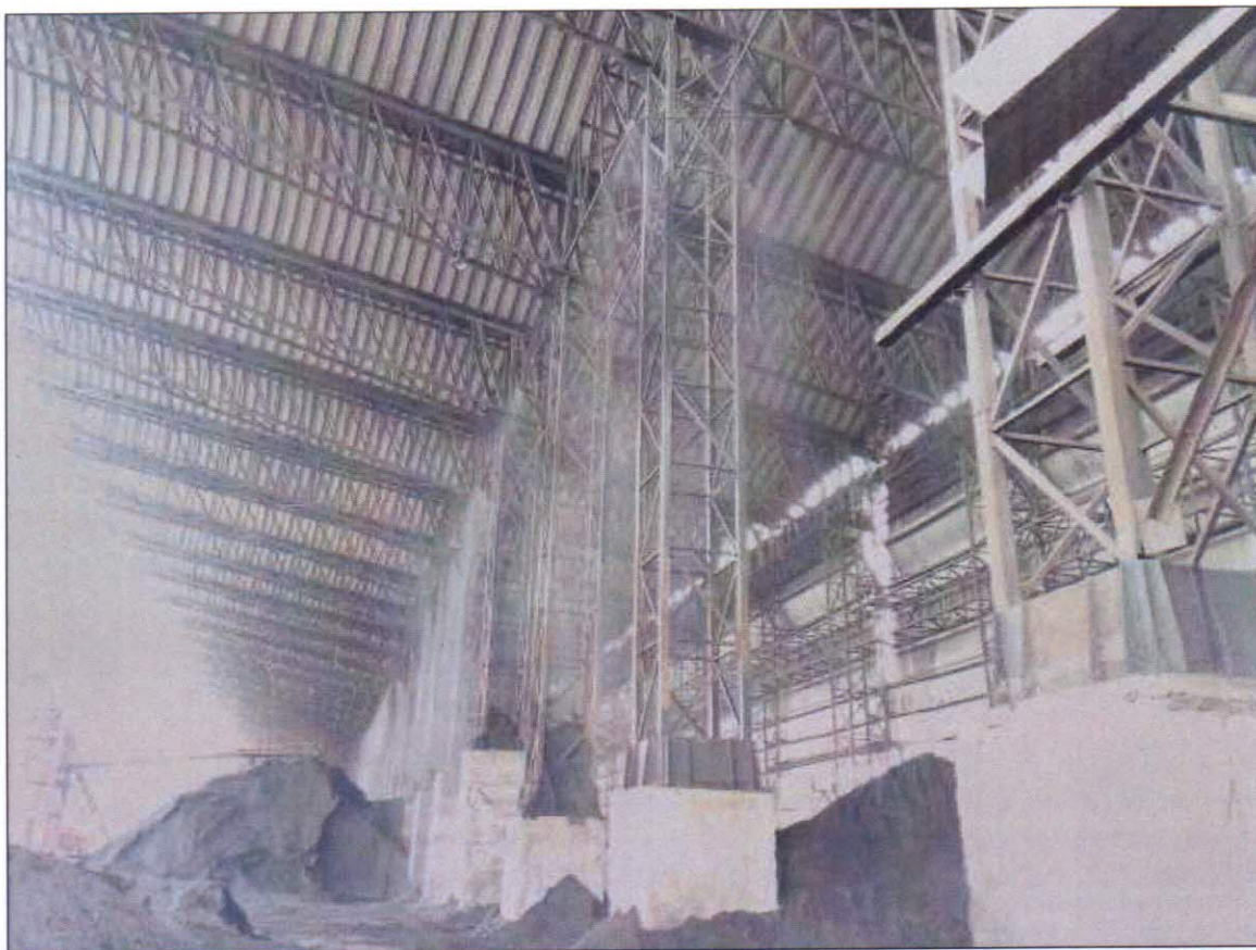
Water Sprinkling System at Monsoon Shed
