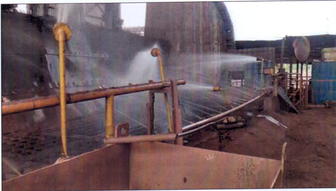
Water sprinkling system at Wagon Tippler unloading system
