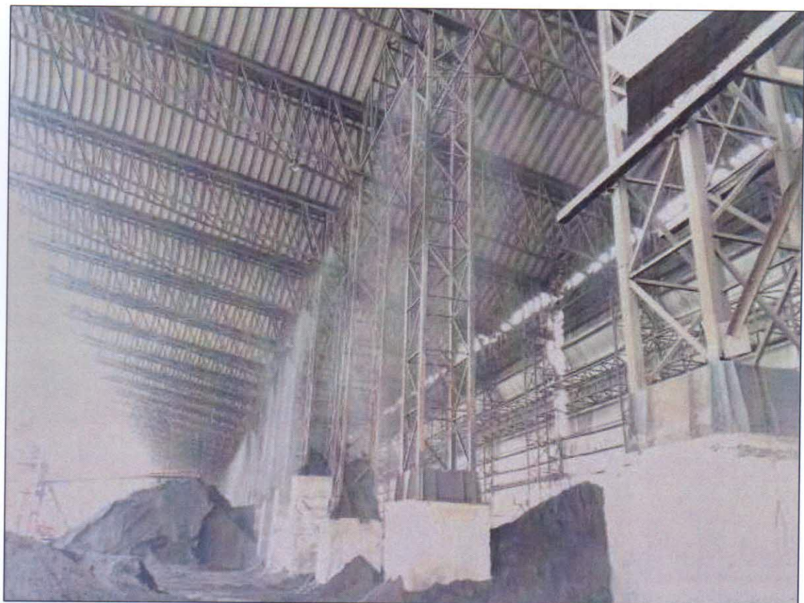
Water Sprinkling System at Monsoon Shed
