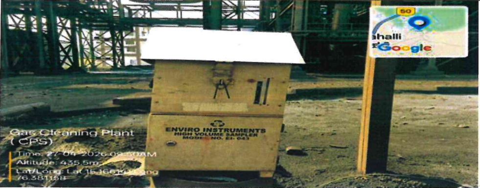
Blower Area Time: 27-04-2026 09:47AM Altitude: 435.5m Lat/Long: Lat 15.166141 Long 76.381158
