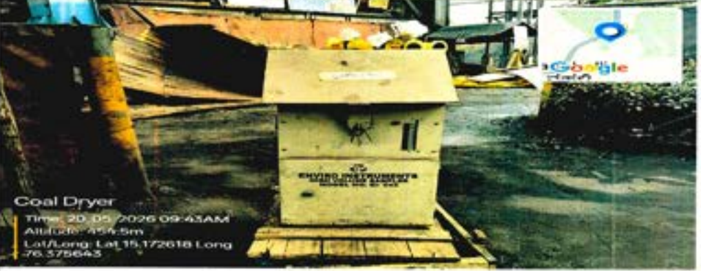
SID-3 Near Coal crusher Time: 19-05-2026 09:41AM Altitude: 444.3m Lat/Long: Lat 15.173697 Long 76.578576
